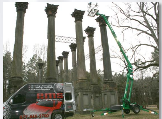
With the columns exceeding 44 feet, EMS used a lift to 3D scan the intricacy of column capitals.
